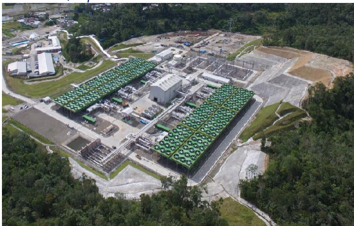
Sarulla Geothermal Independent Power Producer (IPP) Project
