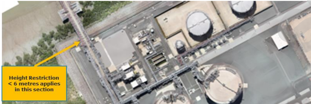
Figure 16 - Jetty Trestle underpass height restriction
