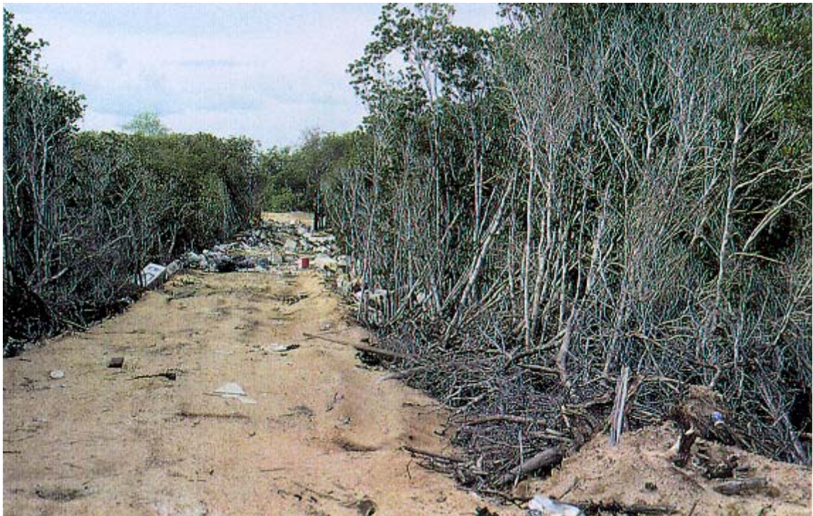
Plate 6 A sand dam placed through mangroves leads to upstream ponding; mangrove death and high numbers of mosquitoes.
