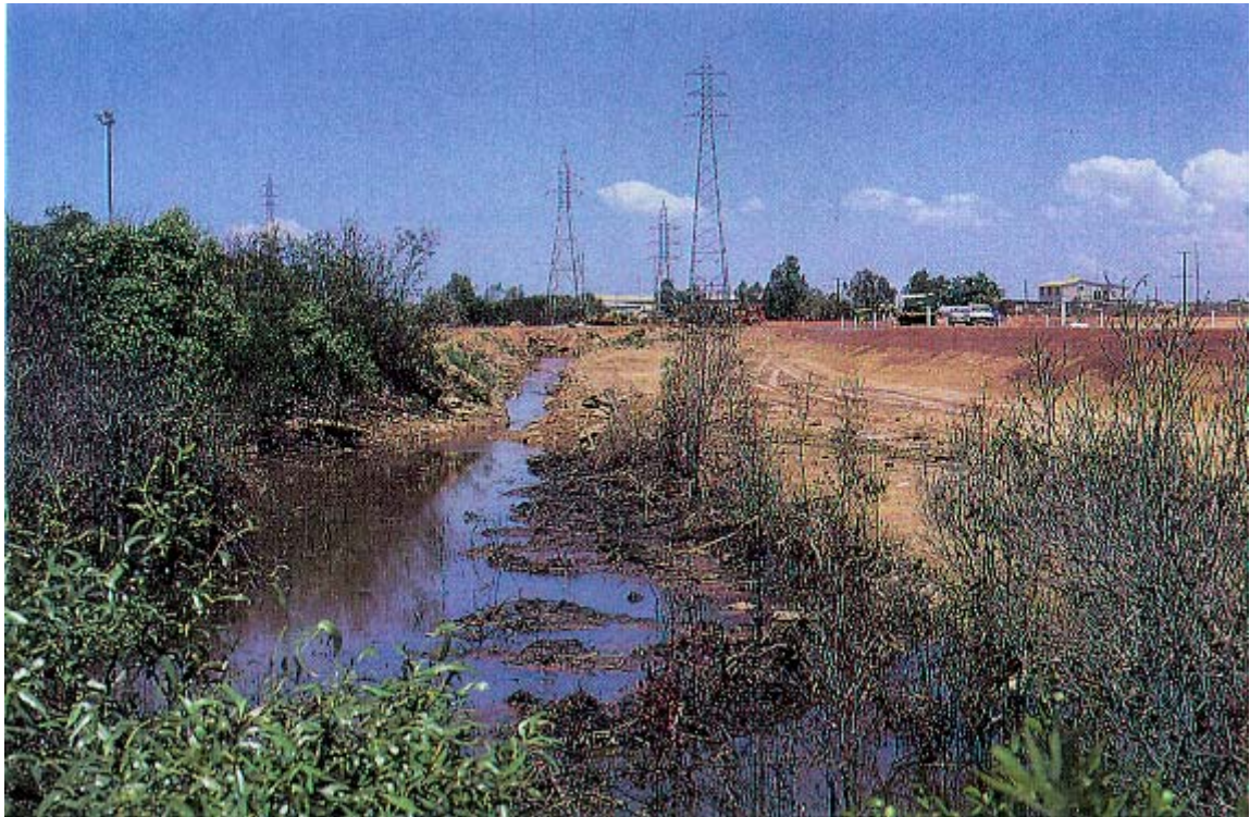
Plate 5 Pooling of stormwater through inadequate drainage creates mosquito breeding sites.
