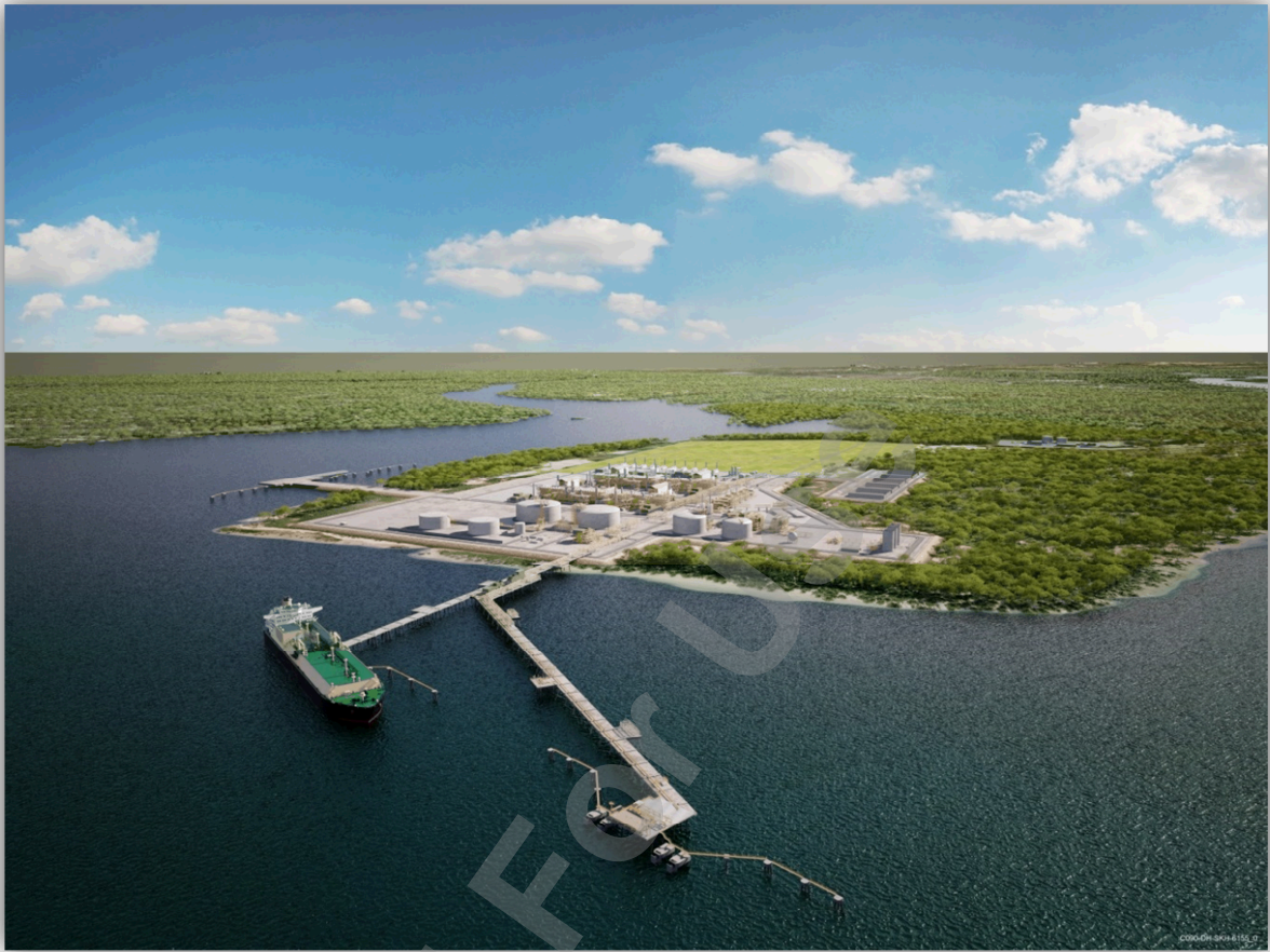
Figure 5 - Ichthys Onshore Facilities
